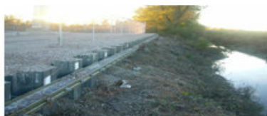
Fig.3 Sea wall made of sheet piles (Fiberglass composite pilings for residential piers and Docks)
