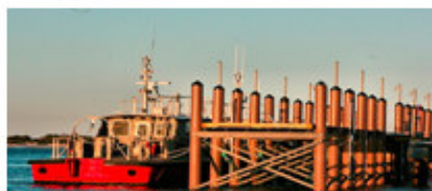
Fig.1 Fiberglass pile (fiberglass composite pilings for residential piers and docks)
